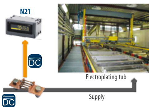
Current measurement in an electroplating plant
